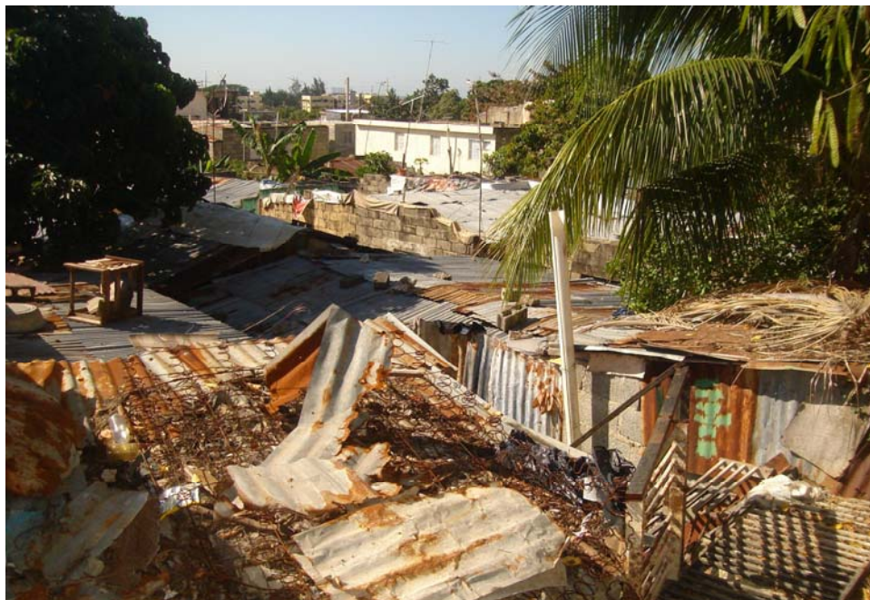
Figure 2. Photograph showing some of the materials that have been used to construct the Luz Consuelo neighborhood Santo Domingo, Dominican Republic.
