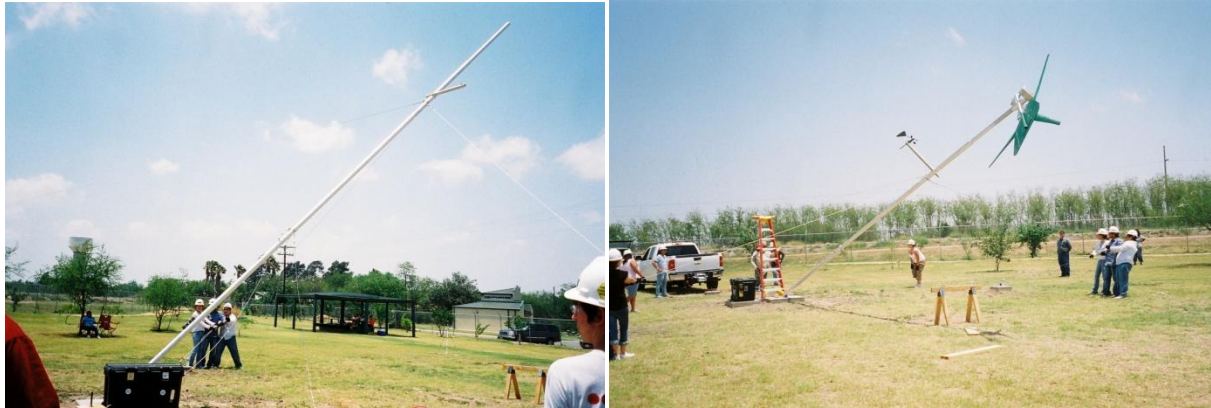
Fig. 12 Students Erecting the 30' Tall Wind Turbine
