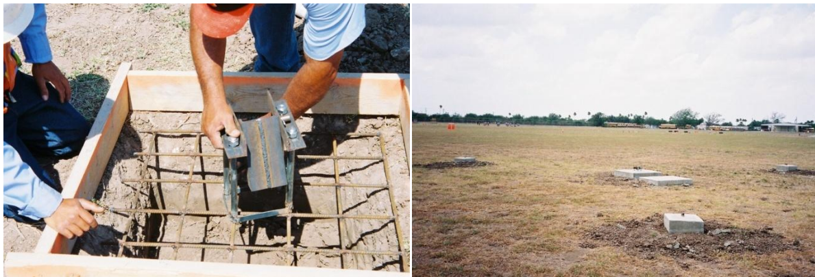
Fig. 11 Preparation of the Base for the 30’ Tall, 100 lbs Wind Turbine
