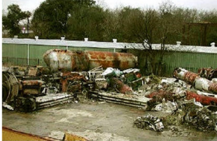
Figure 3. The scene following the explosion
