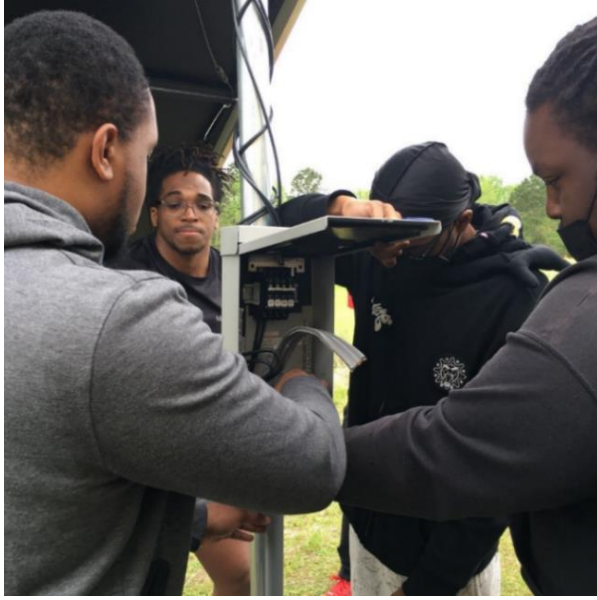
Photo 3. Students completing the wiring for the solar panels
