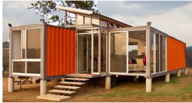
Figure 3. Cargo container home using precast pile foundation 5 .
