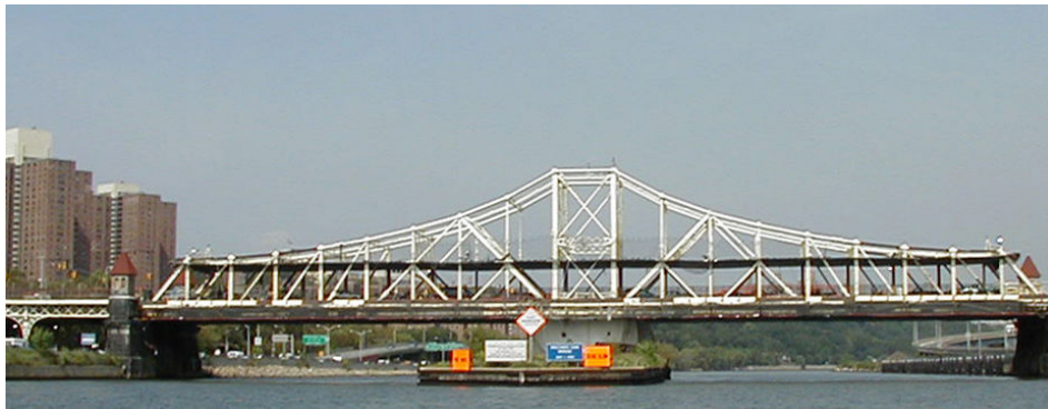
Figure 2: Macombs Dam Bridge
