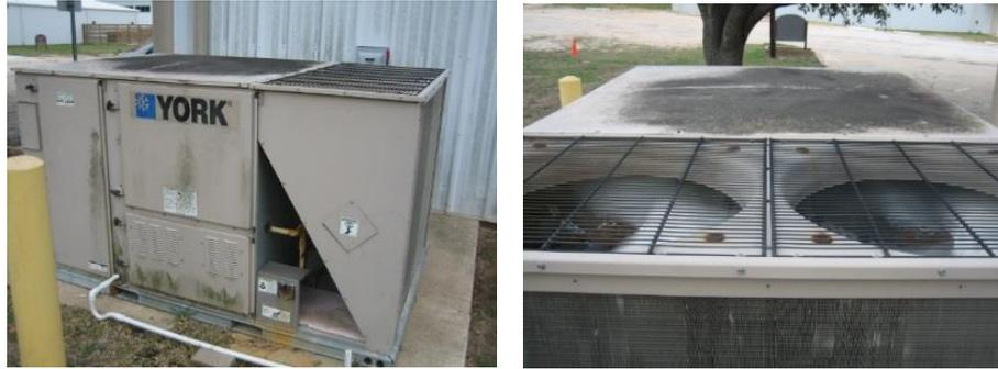
Figure 3. R-410A XP series 6-1/2 ton 60Hz AC Condenser Unit
