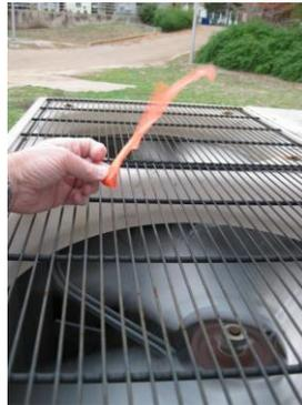
Figure 9. Tape held in area of maximum airspeed showing angle of flow (partially induced by slight ambient wind, but mostly due to rotational flow).
