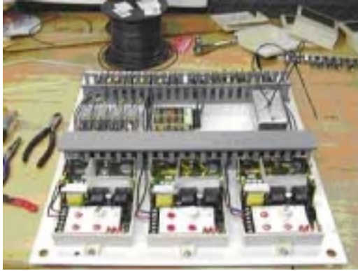
Figure 8. Controller wiring in progress.
