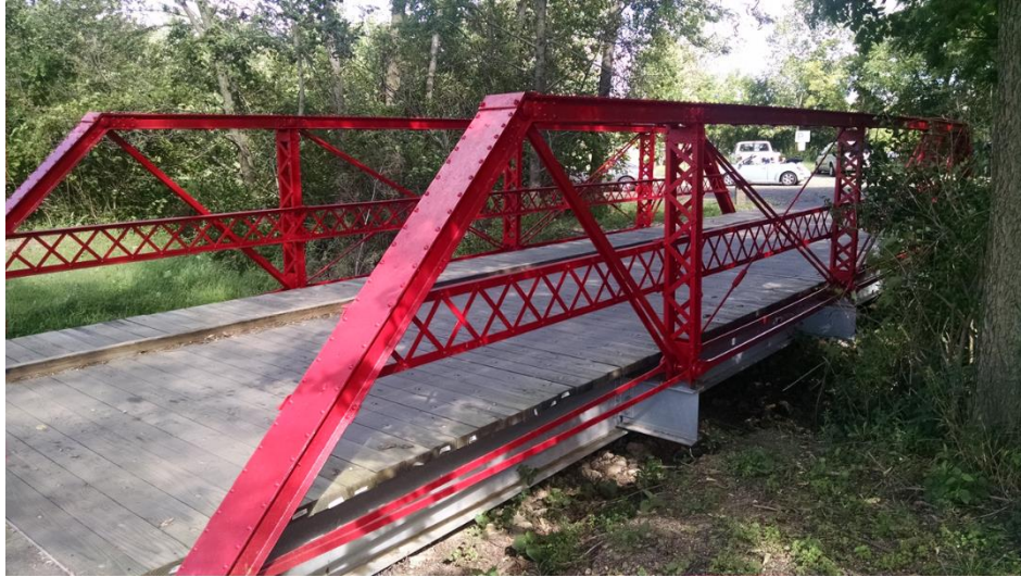
Figure 2 Lucerne Road Bridge in Knox County, Ohio
