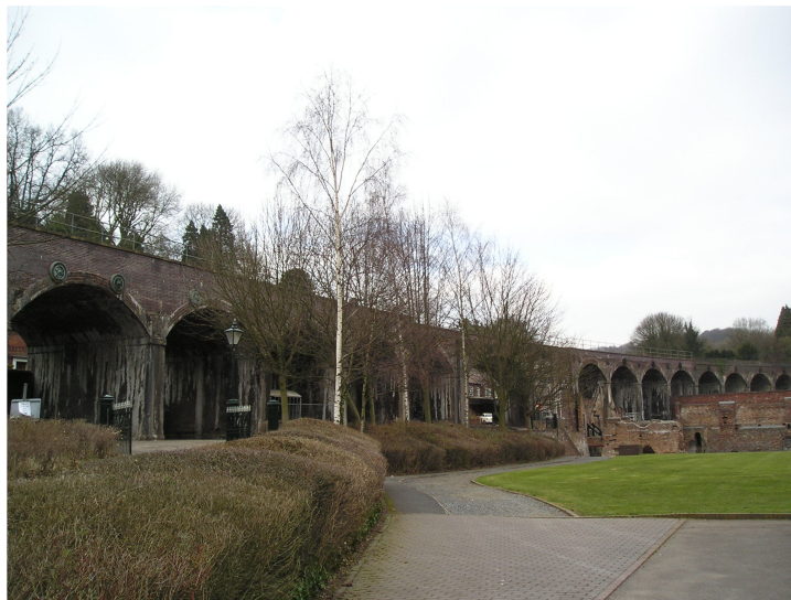
Figure 4. The restored train trestle at Coalbrookdale provided access to the location of the first cast iron foundry in the world.
