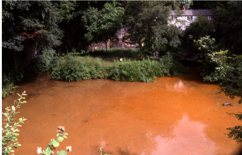
Figure 5. Worsley Delph. The canal arms, left and right center of picture, can be discerned, progressing towards a sandstone cliff. From here, a system of underground canals, eventually totaling 42 miles, was cut on four different levels. The brown color of the water derives from ochre, a hydrated oxide of iron.
