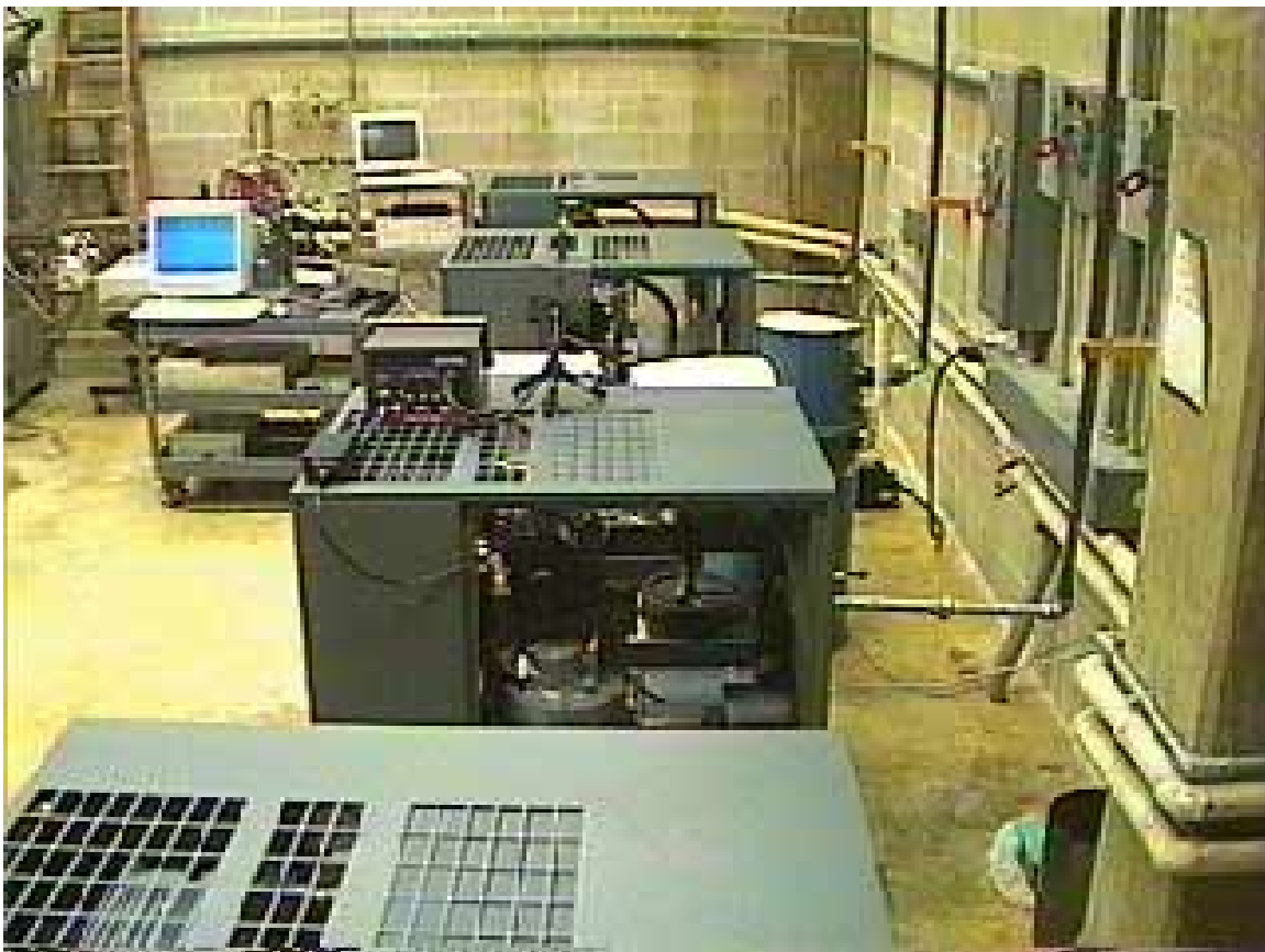
Figure 1. Air Compressor Experimentation Facility.
