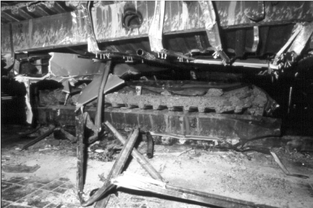
Figure A-2 Failed Walkways
