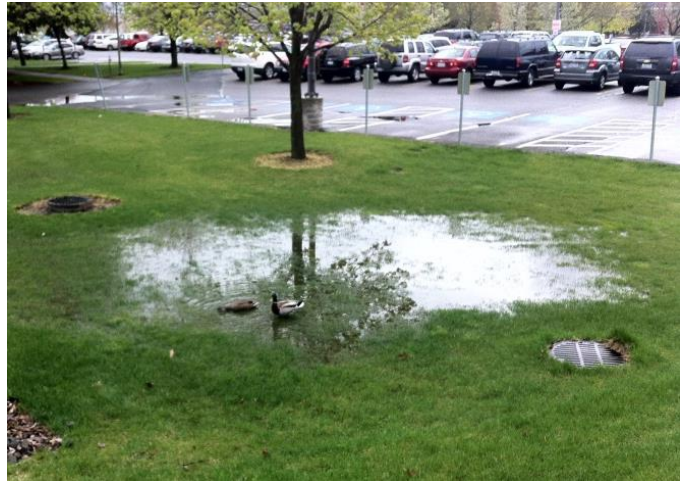
Figure 1. Existing Bio-infiltration Pond
