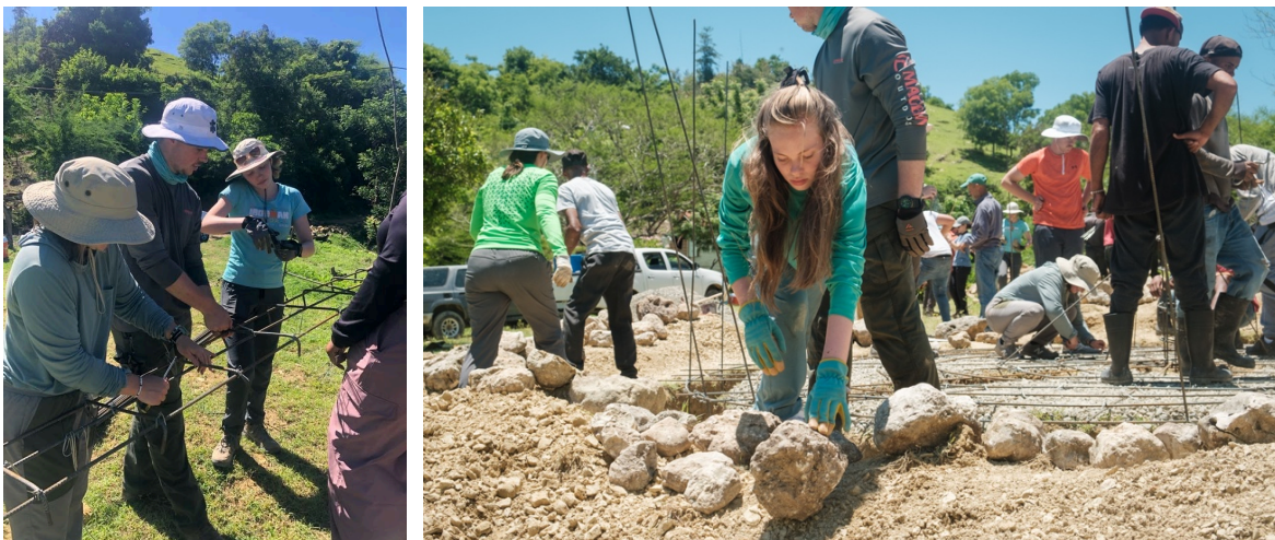
Figure 7: Students tying rebar (left) and constructing the water tank (right)
