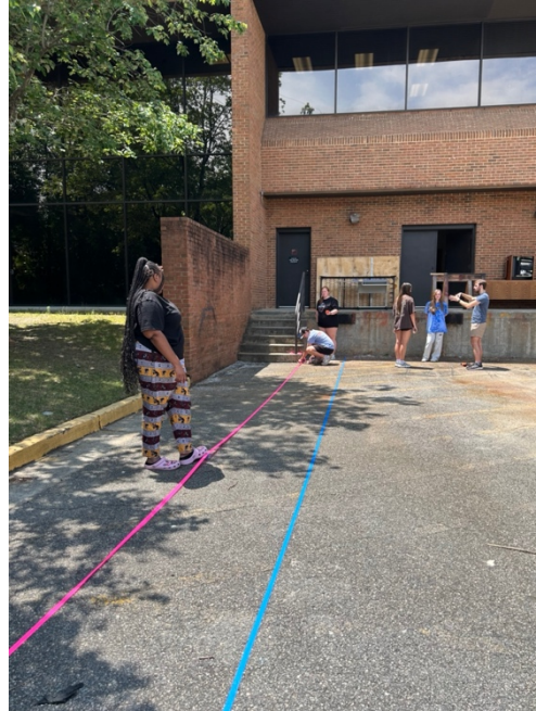
Figure 5. Laying Out a Ramp
