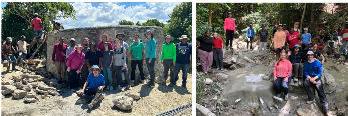
Figure 8: The completed water tank (left) and spring box (right)
