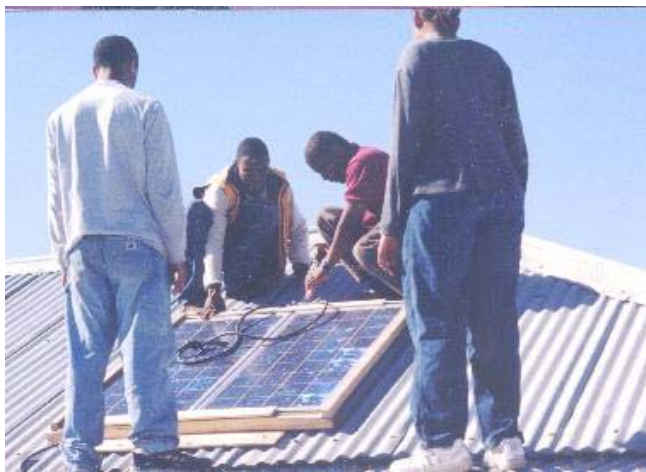
Figure 11: Installing Solar Panels on Roof
