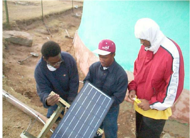
Figure 10: REEP Students Installing Solar Panel
