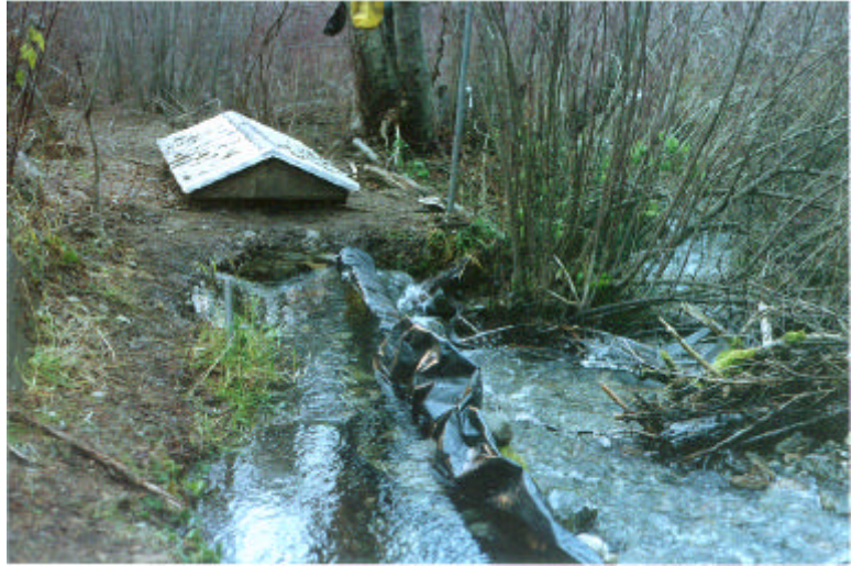
Figure 6. Diversion dam and covered intake box
