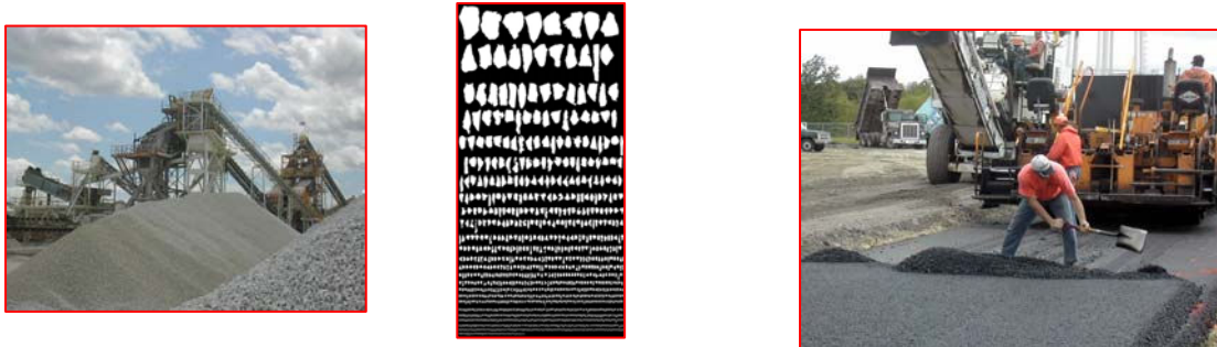
a. Aggregate stockpile b. different aggregate size c. asphalt concrete construction
