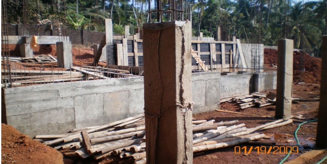
Figure 5: Columns are cured for at least 28 days
