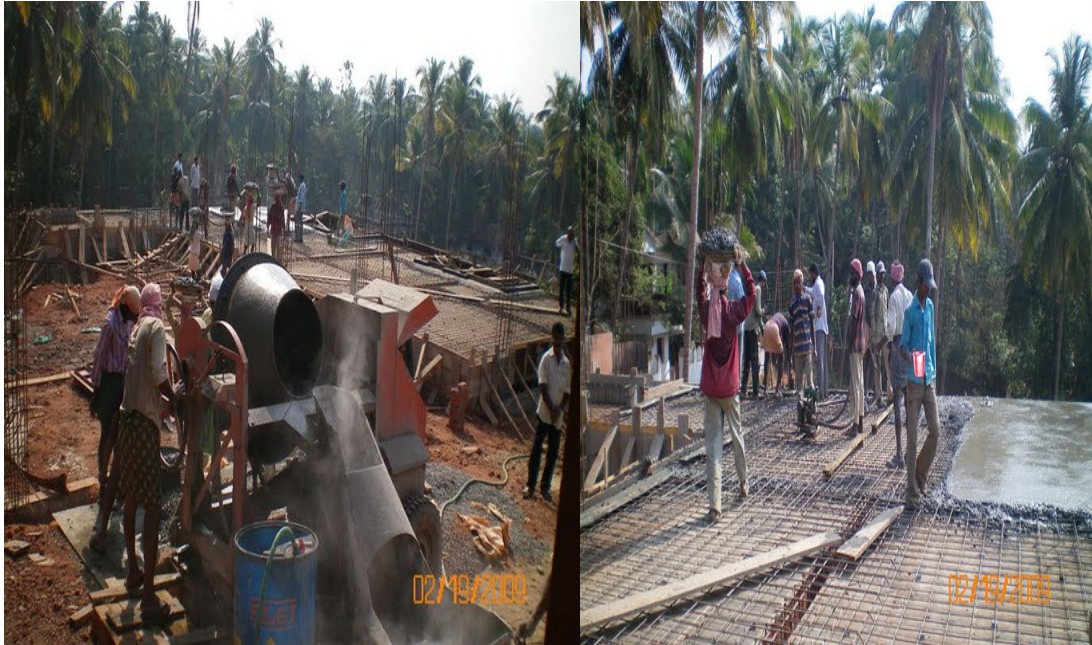
Figure 7: Manual labor working on slab
