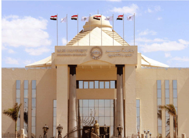
Figure 1. The MUST Administration Building.
