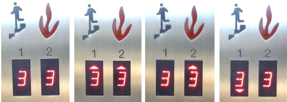
Figure 9: Two elevators at the 3 rd floor: which one is expected to arrive earlier to the 5 th floor?
