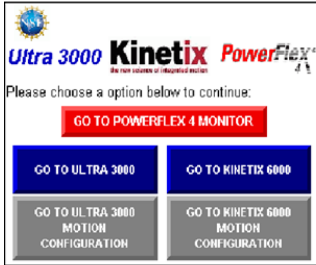
Figure 6: Allen-Bradley PanelView™ Plus 600 HMI Main Screen
