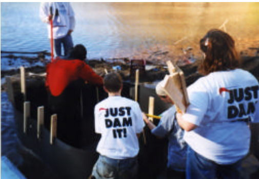
5—Circular PVC coffer dam changes shape
