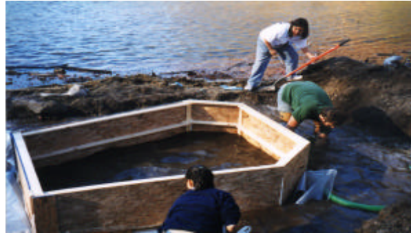
2—Installing the “Coffin Dam”
