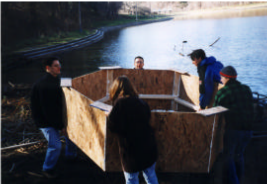
3—Installing a hexagonal coffer dam
