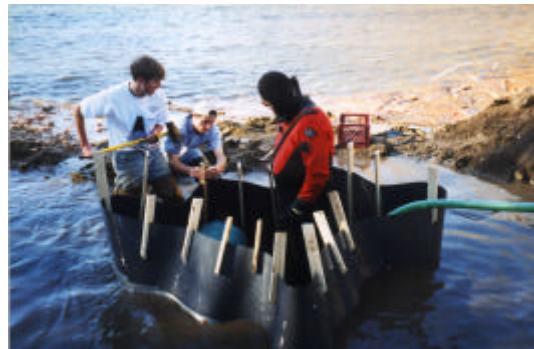
6—PVC “amoeba” is dewatered
