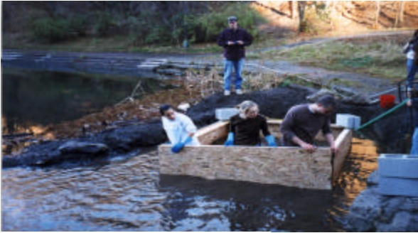
1—Installing a coffer dam
