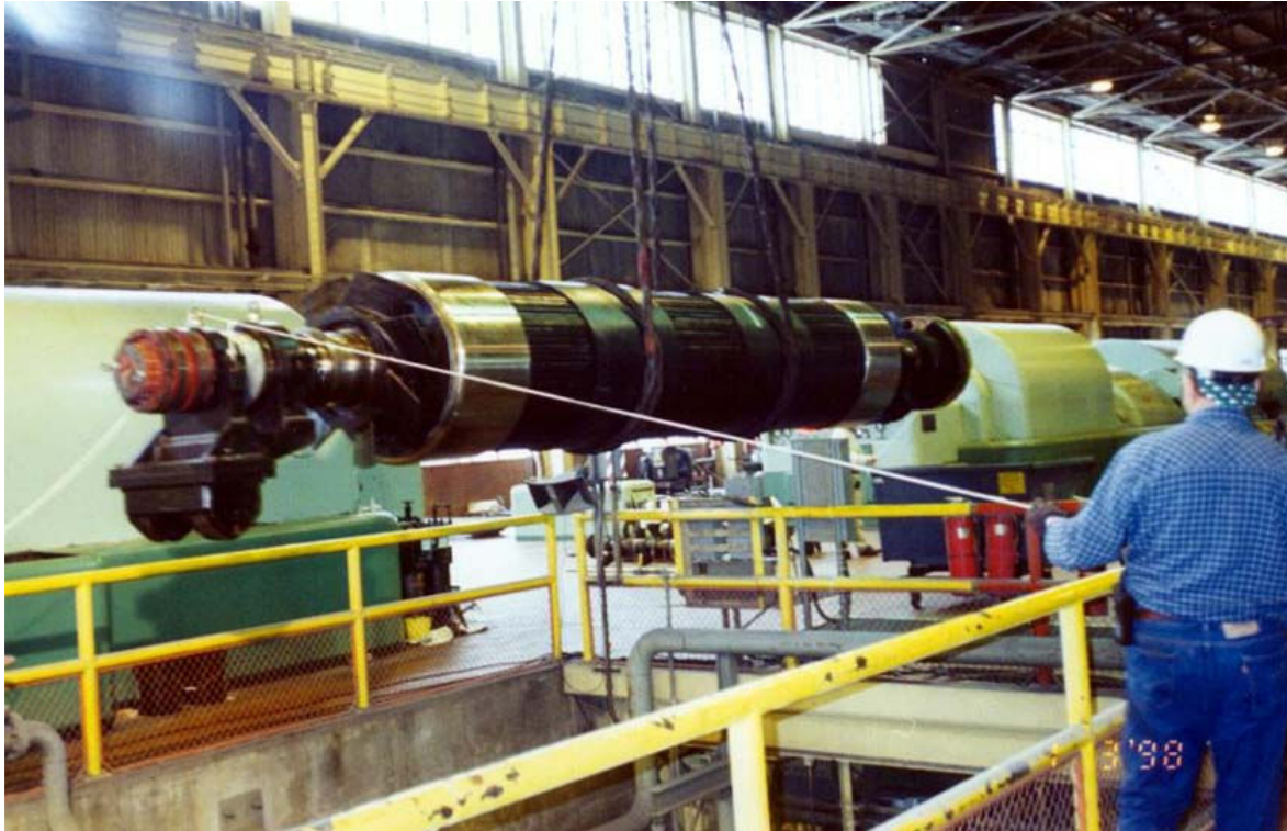
Figure 3: Dismantled Turbine generator unit
