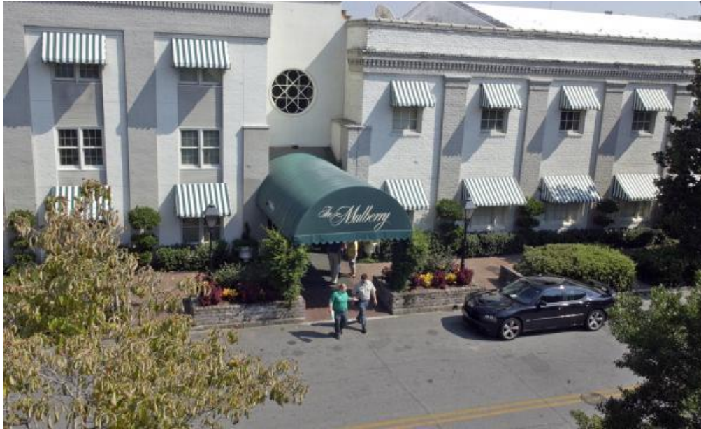
Figure 1. Hotel renovation and restoration
