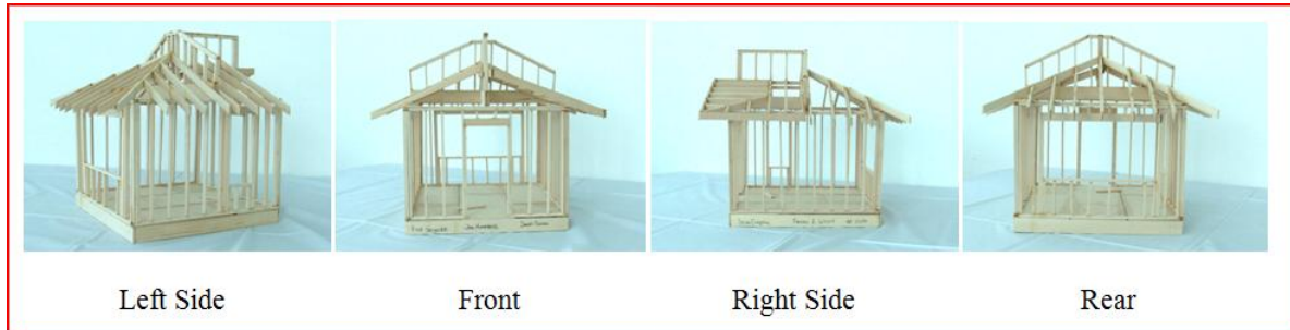
Figure 3 – Framing Cube Stick Build Model
