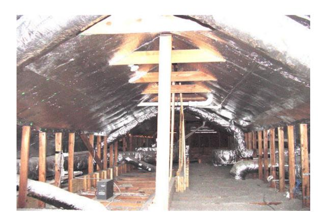
Figure 7, Radiant Barrier Application
