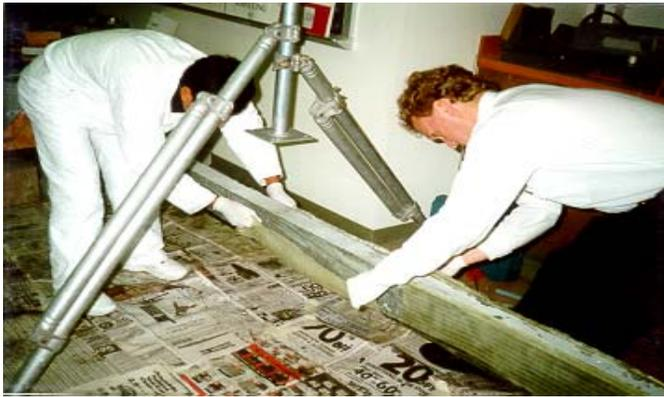
Figure 4 – Students applying fiberglass-reinforcing mesh to beam
