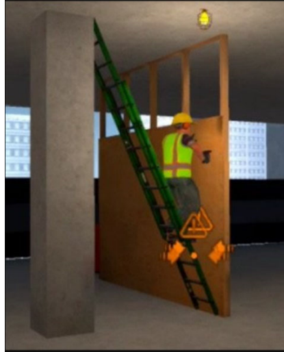
Figure 4: Man on Unstable Ladder (ITI Construction Hazard)
