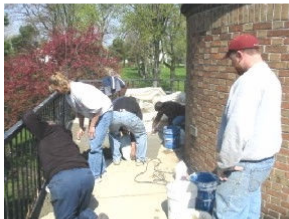
Fig. 8. Repairs being made to concrete deck.
