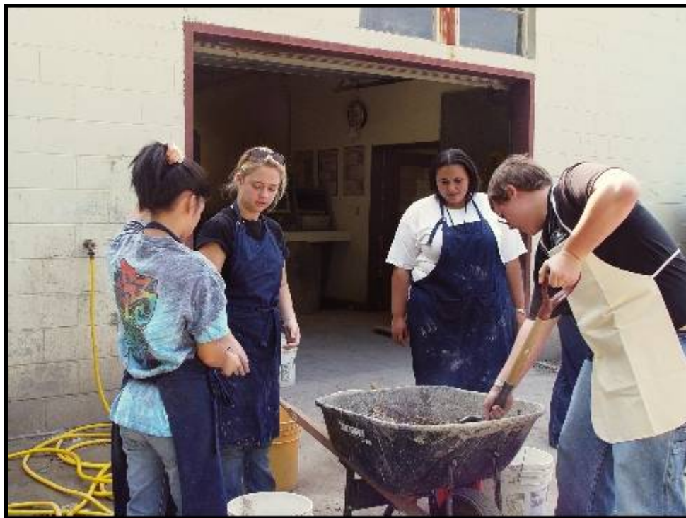
Figure 3: Students Mix Concrete
