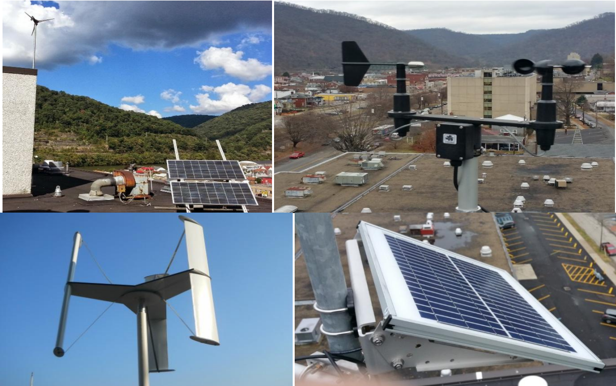
Figure 19: Residential wind turbines (both horizontal and vertical wind turbines), solar PV units, and weather station installed on the roof of the engineering building
