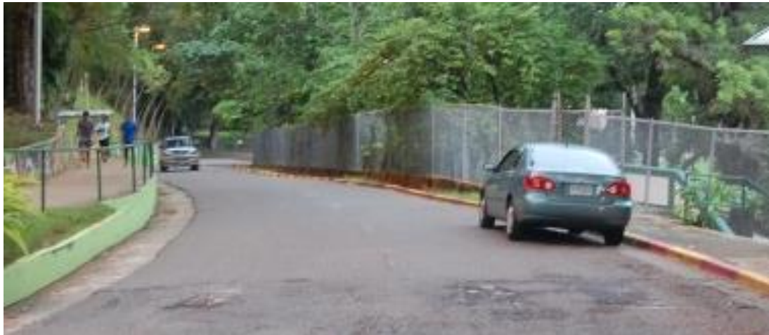
Figure 1. Photo of Road for Module 1.
