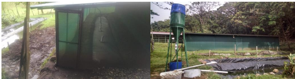
Figure 2: Photo of the agricultural waste treatment system that includes two tubular anaerobic digesters, one struvite precipitation reactor, and four lagoons.
