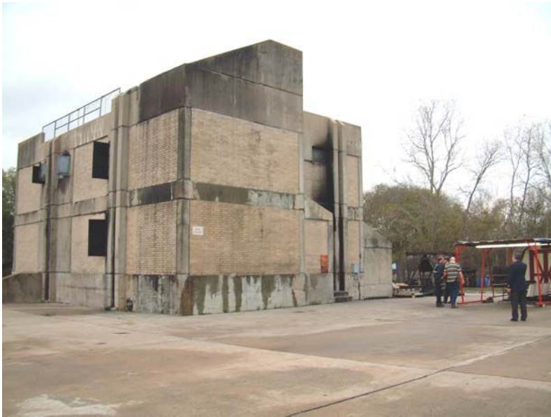
Figure 2. Houston Fire Academy burn house
