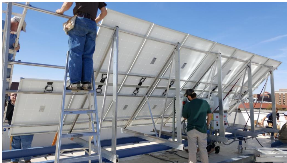
Figure 4. Installation of solar photovoltaic array by students, faculty, and staff.
