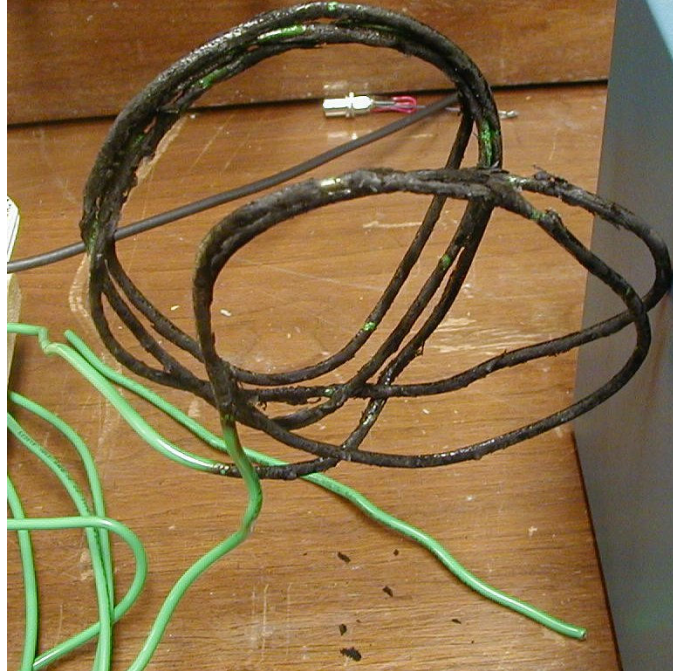
Figure 7. Insulation charred with a propane torch.
