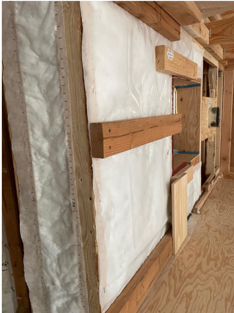
Figure 1. Image of insulation used in integrated truss systems. Photo by Todd Nicewonger, 2022.
