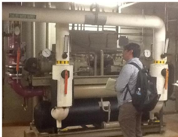
Figure 13. Students Recording Specifications from a Chiller
