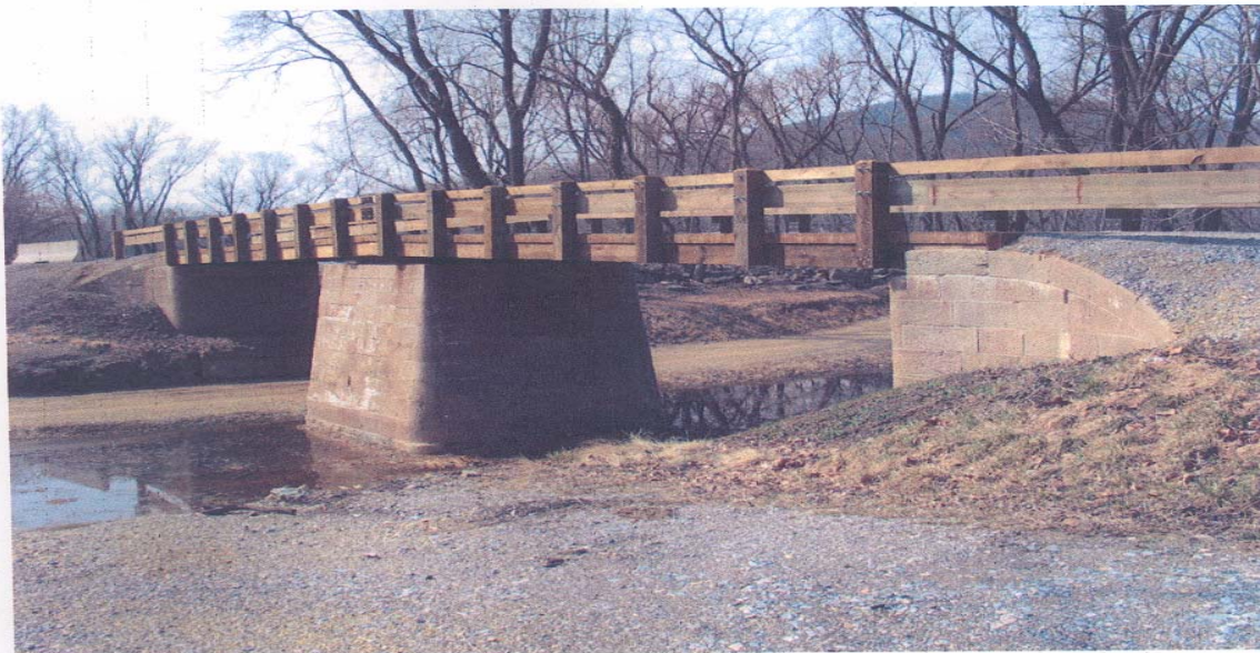
West (Upstream) Side
