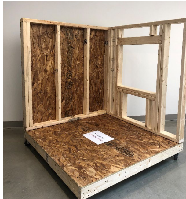
Fig. 2 Residential house frame demonstration.
