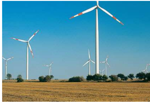
Figure 2. Typical Vestas V82 Installation [18]
