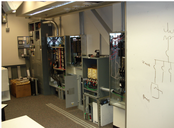
Fig. 1, Complete replica of an electrical distribution system in a classroom.
