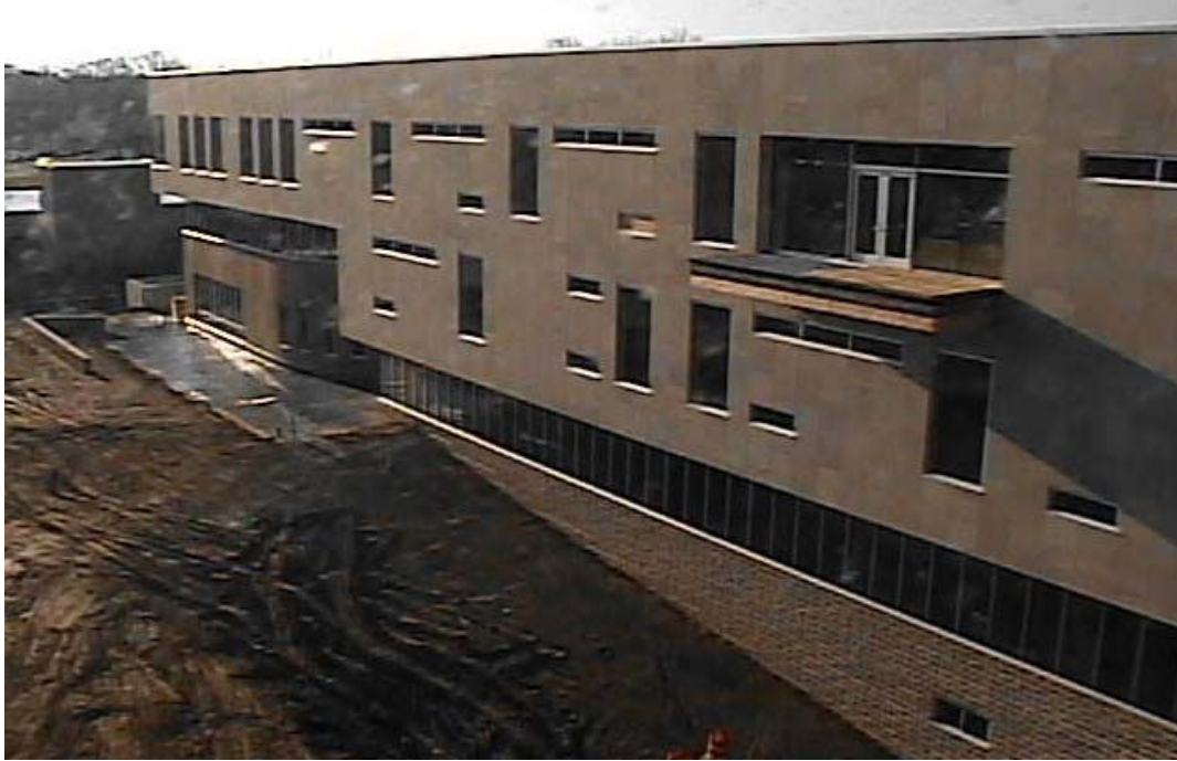
Figure 3: Photo from Construction-Cam of the Business and Engineering Building
