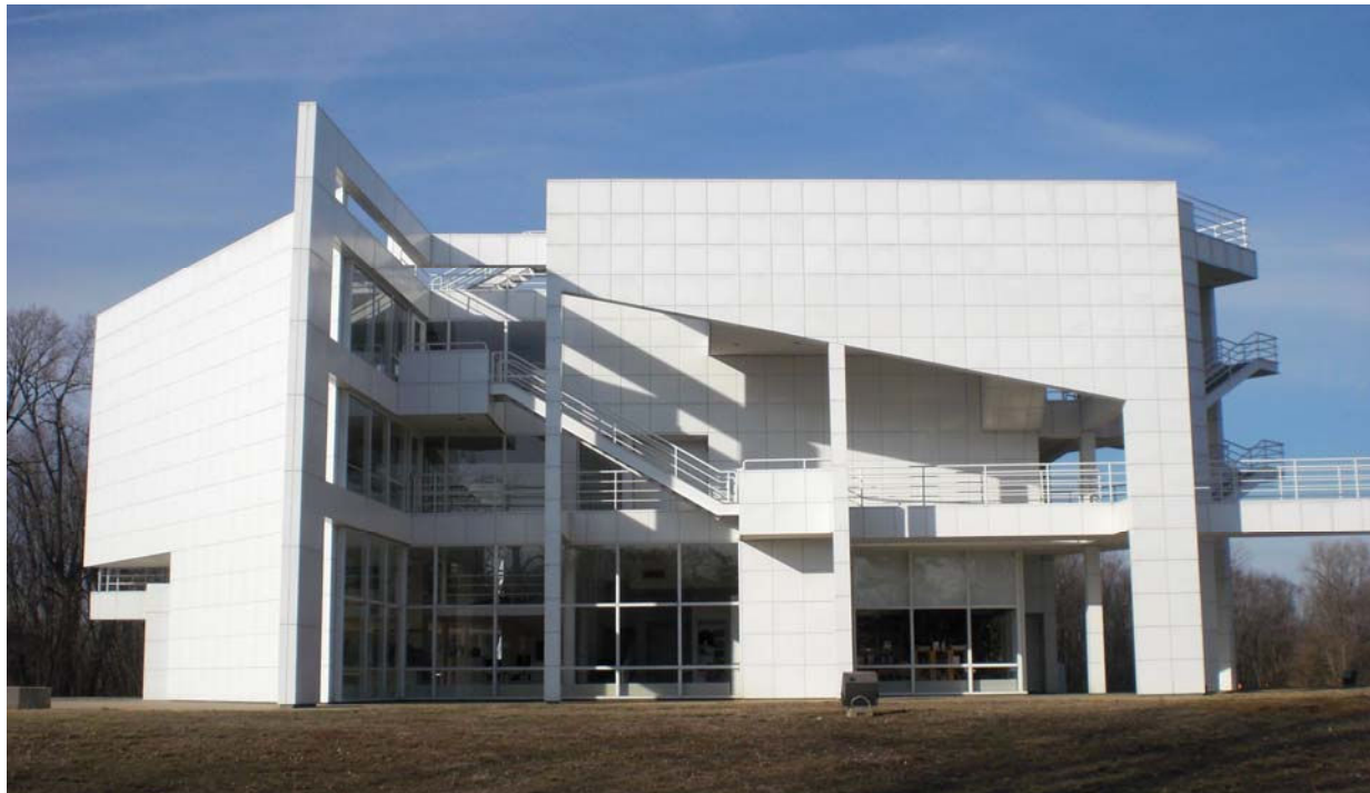
Figure 2: Photograph of Atheneum building showing southern exposure
