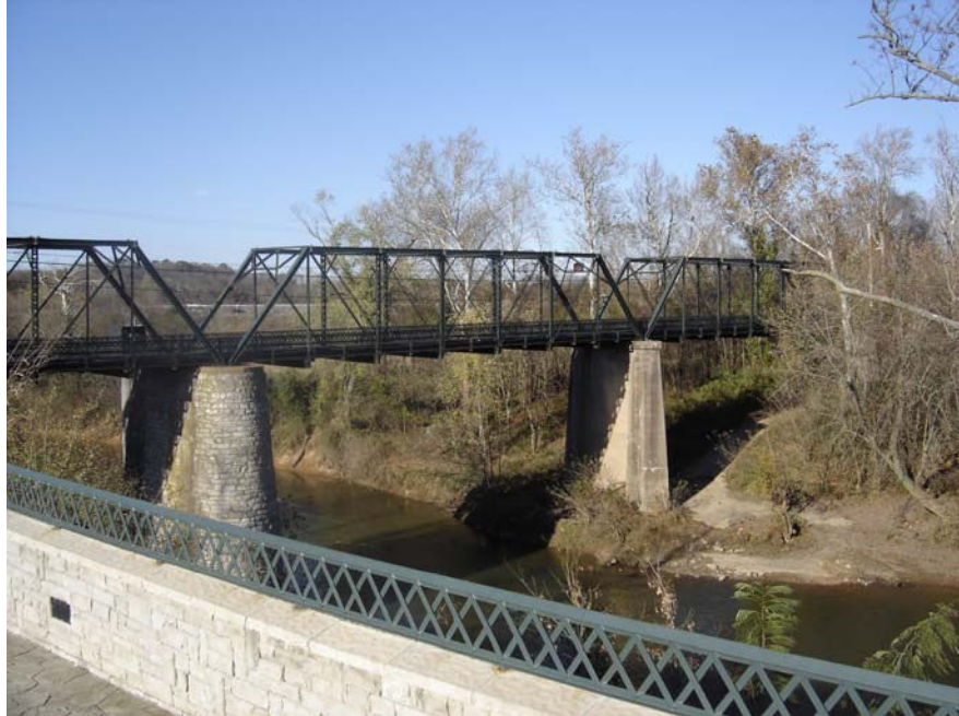
Figure 2: College Street Bridge
