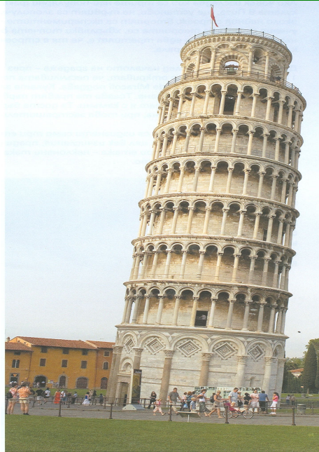
Fig. 1: The Leaning Tower of Pisa
