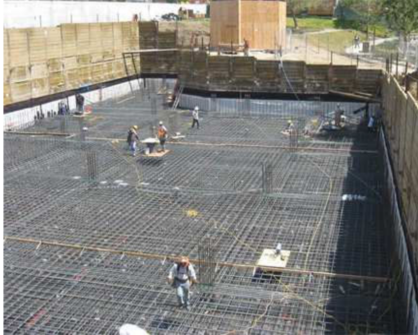
Figure 5: Raft foundation
