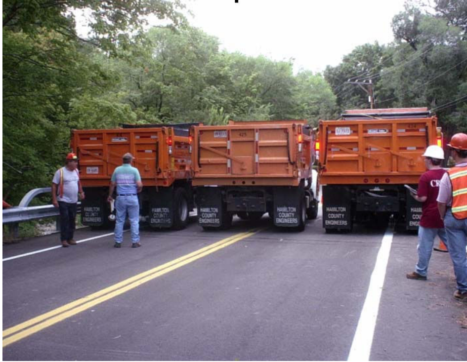
Figure 3. Positioning the Trucks on the Bridge Deck for Testing
