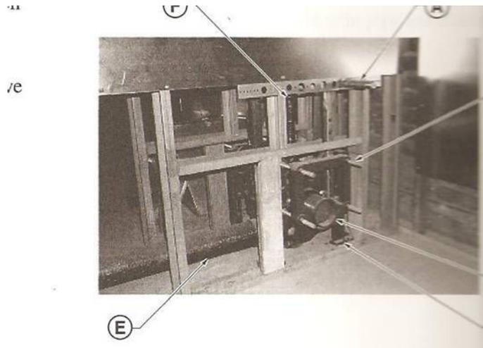
Figure 2: Water Closet Carrier and Fitting<sup>2</sup>
