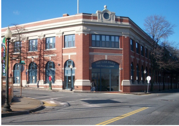
Figure 12 Former car barn at Weld and Purchase St, New Bedford, 2012
