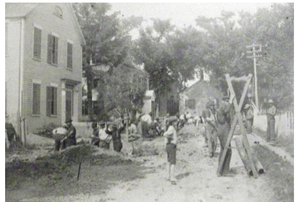
Figure 17 Construction on Church St in Mattapoissett [7]
