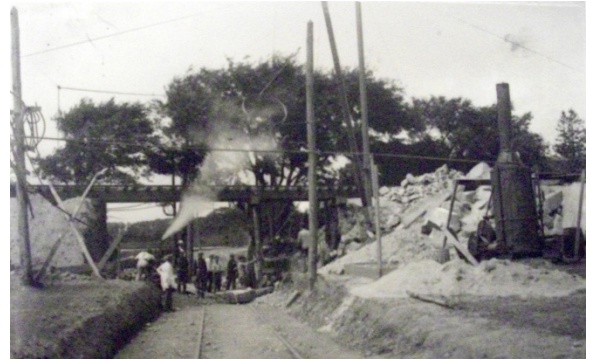
Figure 16 RR Underpass at Mattapoissett [7]
