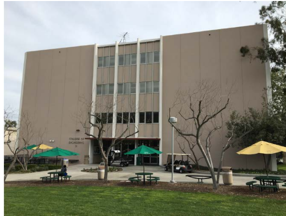
Figure 1: North elevation of five-story building
