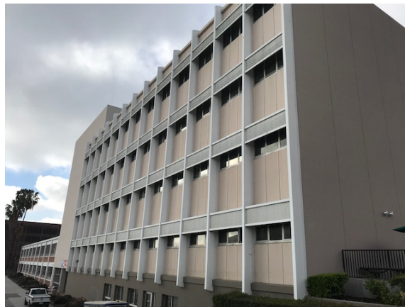
Figure 2: East elevation of five-story building
